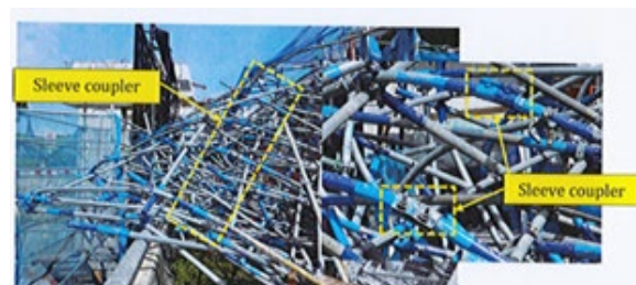
Figure 9. Position of sleeve coupler
