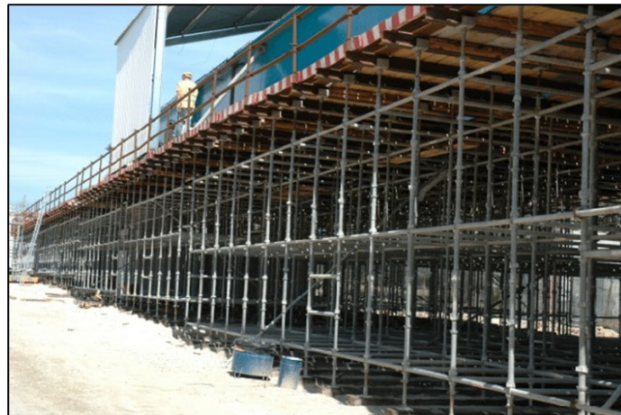
Figure 8. Modular scaffolds used as falsework
