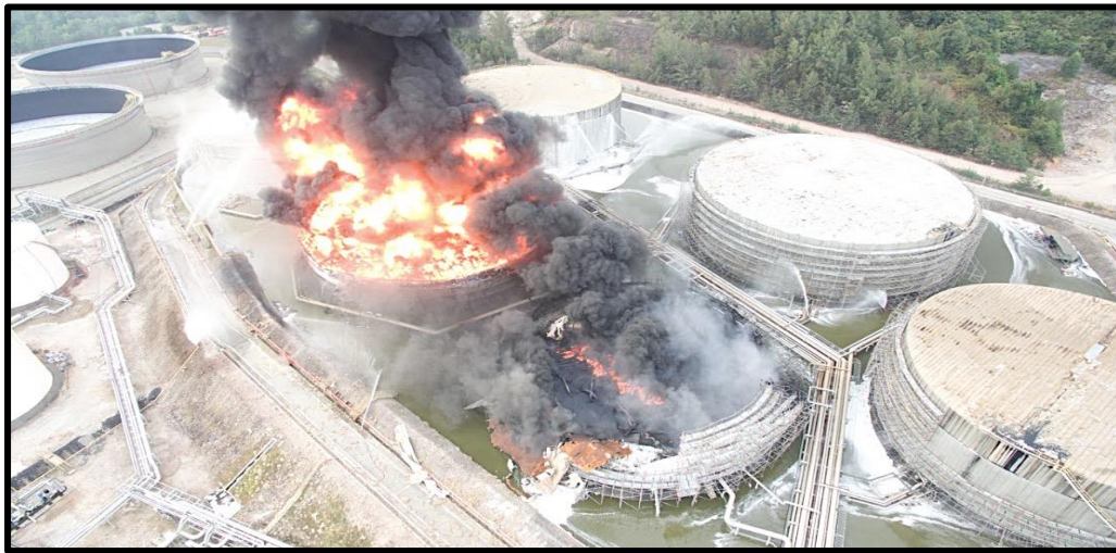
Figure 1: Fire and Explosion –Atmospheric Storage Tank
